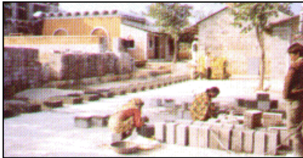
Concrete block production yard
