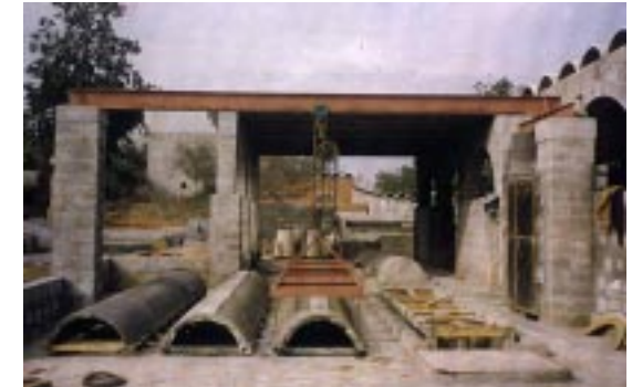
Ferrocement channels production yard
