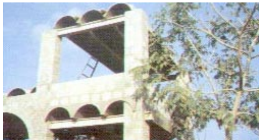
Ferrocement Channels as an intermediate floor
