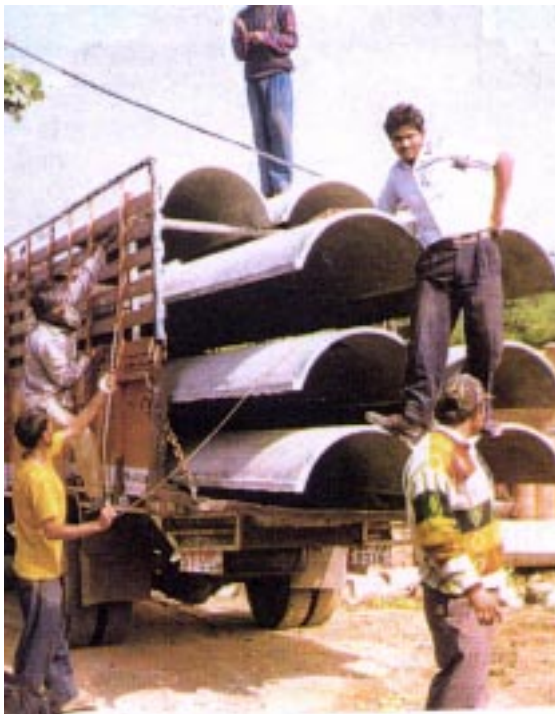
Transporting ferrocement roofing channels
