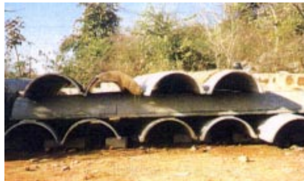
Profile of Ferrocement Roofing Channels
