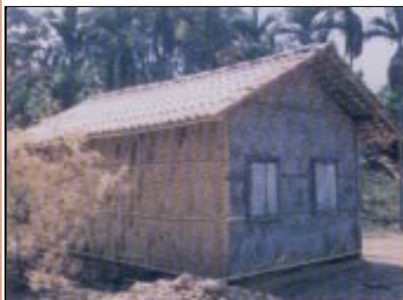
Upgradation of house using Micro Concrete Roofing technology in Tura, Meghalaya
