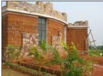
Figure 16 : Building construction using Laterite and sand stone in Bhubaneswar
