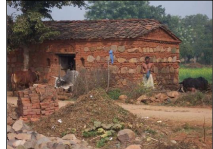
Figure 12 : Semi-pucca house with composite mud and stone masonry wall and country tile roof
