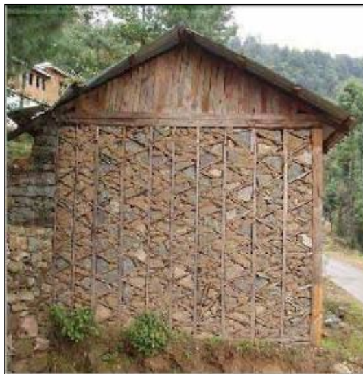
Figure 8: Traditional Dhajji wall construction in Himachal Pradesh
