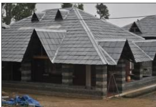
Figure 7: Stone slate roofing
