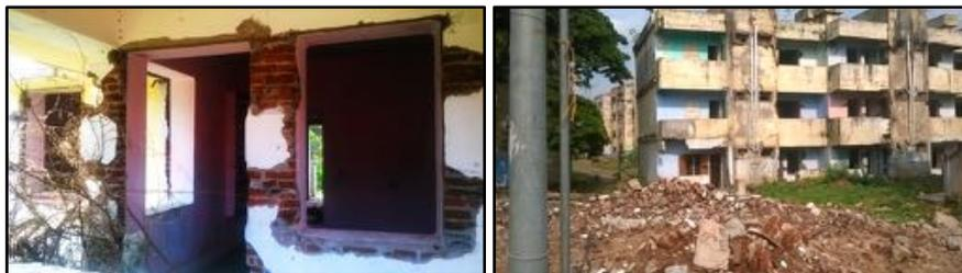
Window and Door Frames Being Removed Before Demolition (Left)
