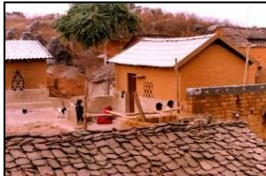
Figure 12: MCR tile roof in semi-arid Bundelkhand as an alternative for burnt clay country tiles
