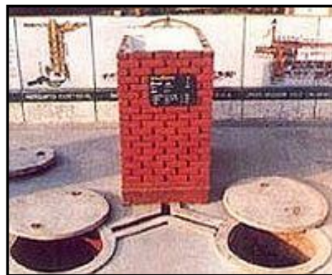
Figure 26: Twin pit toilet
