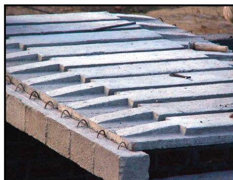
Figure 15: Precast planks and joists (to be finished with in-situ concrete to finish the roof)
