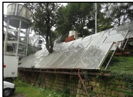
Figure 33: Evacuated tube type solar thermal collectors at a hospital in Dharmsala, Himachal Pradesh
