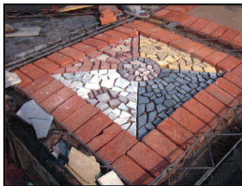
Figure 14: Funicular shell – various small shell segments can be cast on a grid of beams
