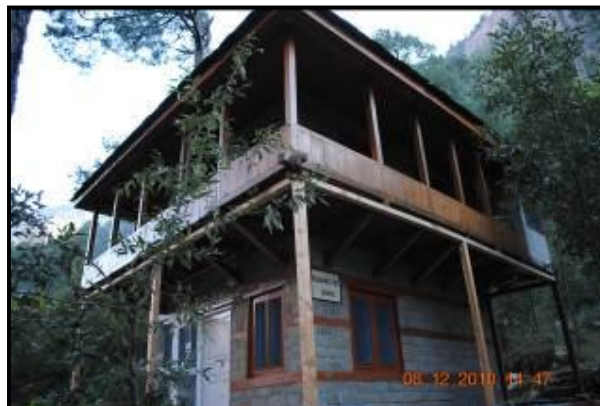
Figure 18: Traditional composite construction of timber frame and masonry in Himachal Pradesh
