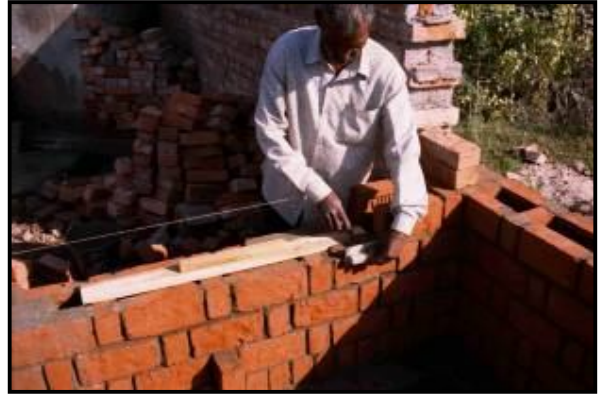
Figure 1: Rat-trap bond wall construction – cavities are left in the wall by a typical arrangement of bricks
