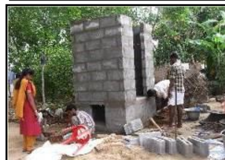
Figure 27: (Above) Ecosan toilet on a raised platform with waste storage below (Below) Ecosan pan for waste separation designed by Biome
