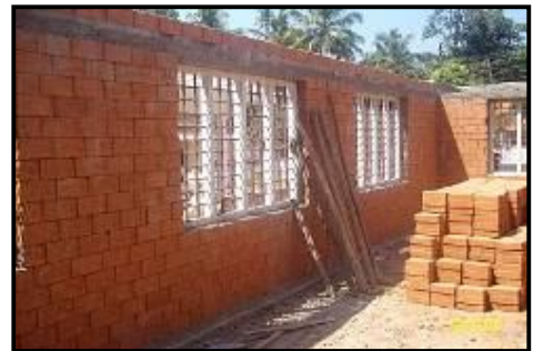
Figure 8: Interlocking laterite blocks for wall construction
