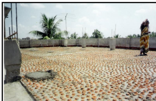
Figure 24: Inverted earth pots on roof
