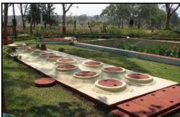
Figure 28: Anaerobic baffled reactor and root zone treatment module in the DEWATS system
