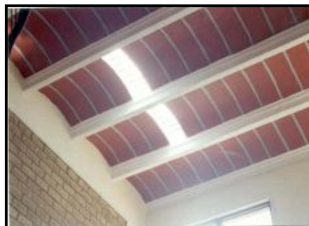
Figure 16: Precast arch panels in community building (above), view of the ceiling
