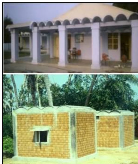
Figure 13: Ferrocement roofing channel roof in an institutional building (above) and disaster resistant Core house in coastal Orissa
