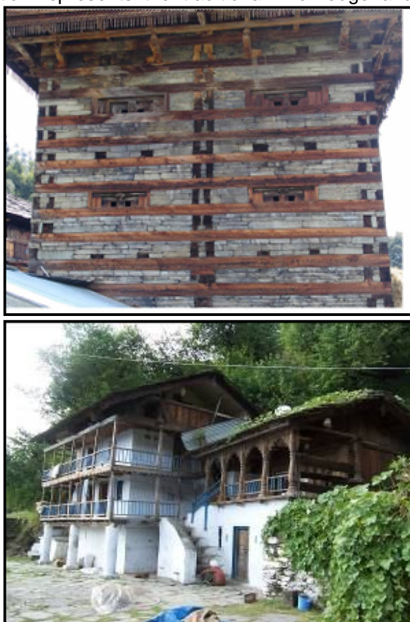
Figure 20: Koti Banal architecture – Wooden logs as ring beams between layers of stone, external verandas resting on massive columns
