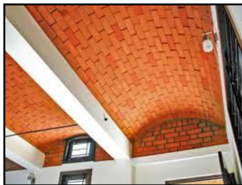
Figure 17: Jack arch roof with burnt clay bricks
