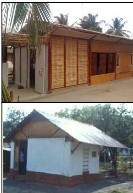
Figure 19: Bamboo frame and cladding for a community building (above) A bamboo prototype house developed by Wondergrass
