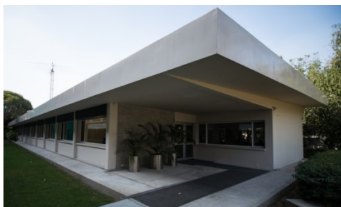
Picture 1: The SDC building at the Swiss Embassy in Delhi having AAC blocks made of LC 3
