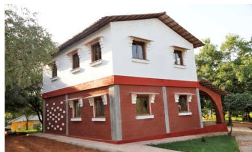
Picture 2: Building in TARAGram Orchha, India made with LC 3 cement
