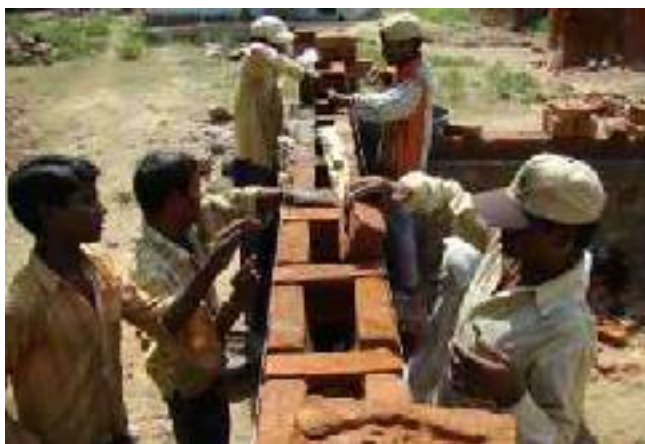
Trained masons at work
