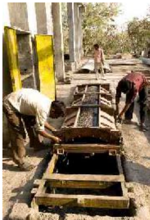
Community workers manufacturing roofing channels
