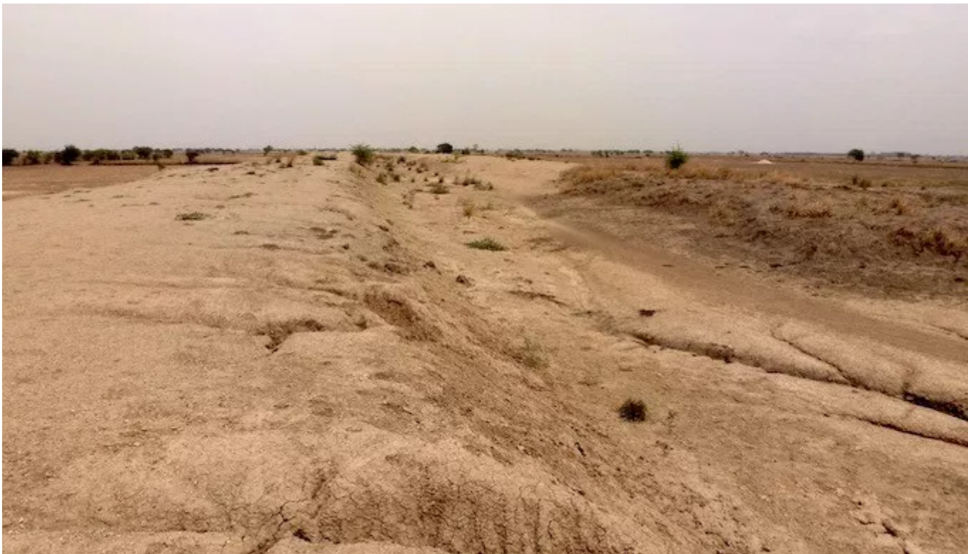
A canal being built to be part of the Ken-Betwa river linking project. Photo: Soumya Sarkar.
