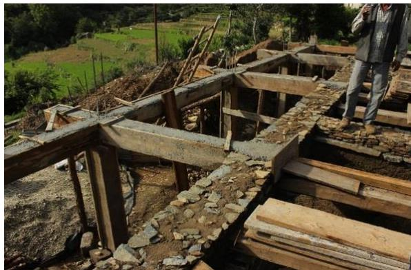
*RCC columns and beams combined with traditional stone masonry in Kamad village*
