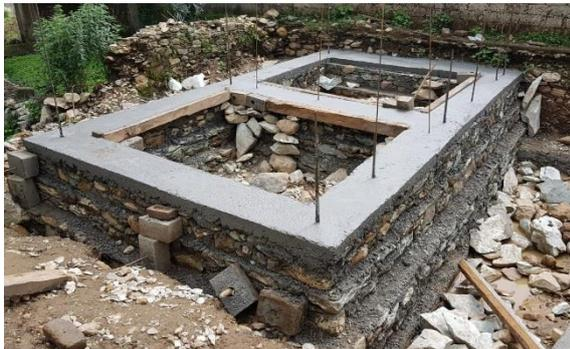
Strip footing in mortar ratio not leaner than, 1:6 is to be provided under all load bearing walls of the structure and all eccentric foundations are to be avoided. The depth of the footing is still a strata with sufficient bearing capacity. It is observed that rocky strata is found at shallow depths of 2-3 feet in most parts of Uttarkashi. A 150mm deep RCC plinth beam is to be provided across the thickness of the walls, for all load bearing walls.
