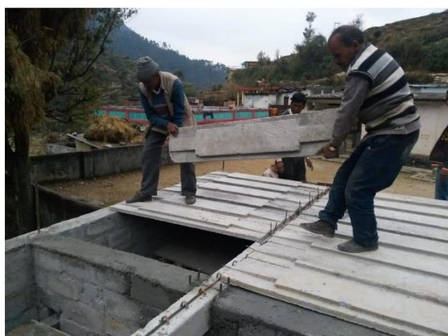
Plank and Joist technology is a modular construction system based on standardized dimensions of planks and joists. The planks are made to standard dimensions and must have at least 50mm bearing on the joists and walls.
