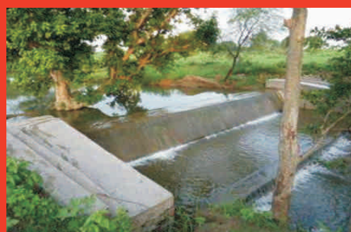
Checkdam built in Govindnagar
