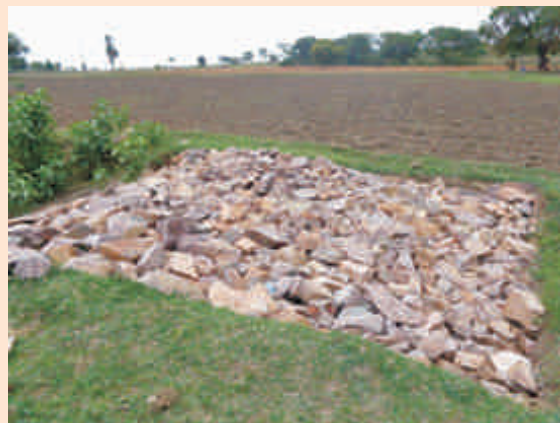
Loose boulder structure for minimizing water and soil run-off
