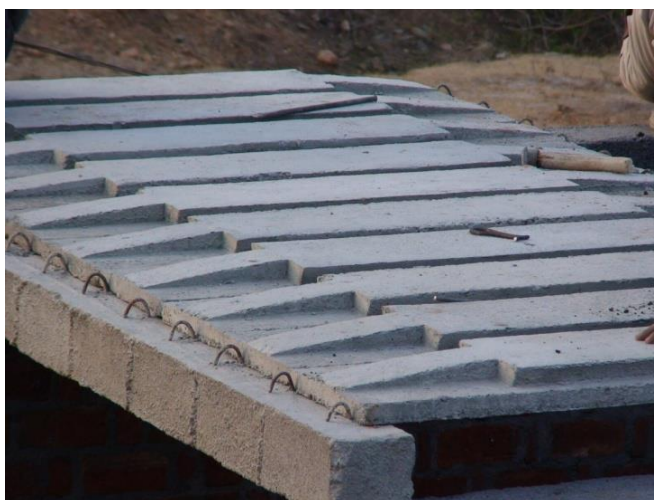
Image of assembled plank and joist roofing technology
