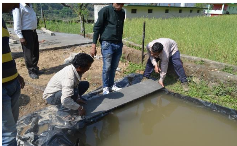
The curing process of plank after 24 hours of its casting
