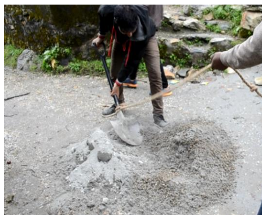
Image of preparation of concrete mix manually
