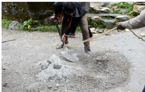
Preparation of concrete mix manually.
