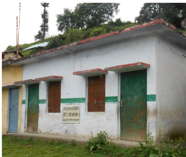
Shift from timber to steel door and window frames Use of timber door window frame sin new construction practices
